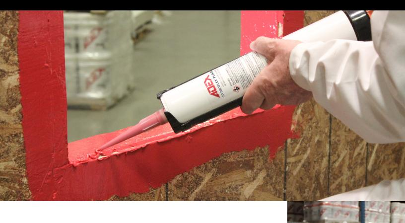
**HYDROFLEX FLASH** is a waterproofing, adhesive, and detailing compound for air barrier applications that combines the best characteristics of silicone and polyurethane. It is a one-component, liquid-applied, Silyl-Terminated-Polymer (STP) material that is easy to gun, spread, and tool to produce a highly-durable, seamless, elastomeric flashing membrane.
